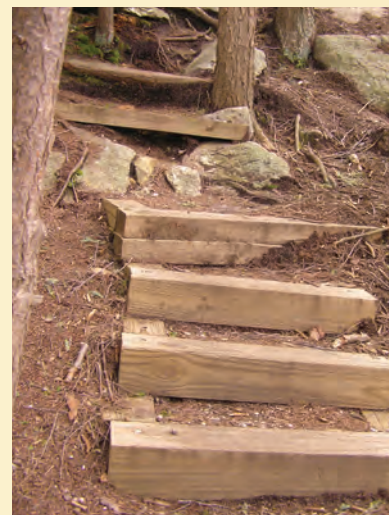
Cribbed stairs on a steep grade improve safety and reduce erosion.
