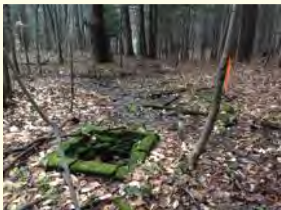
A hand dug well along south border.
