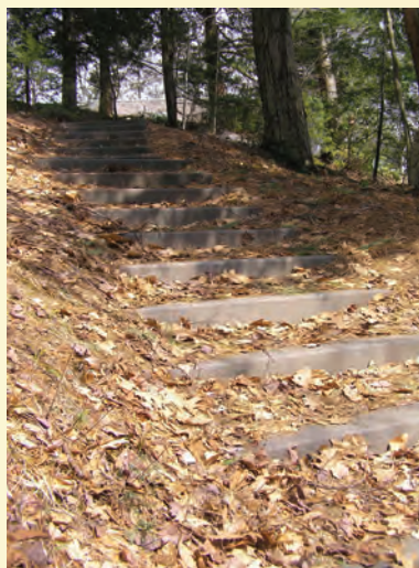
Cribbed stairs on a steep grade improve safety and reduce erosion.
