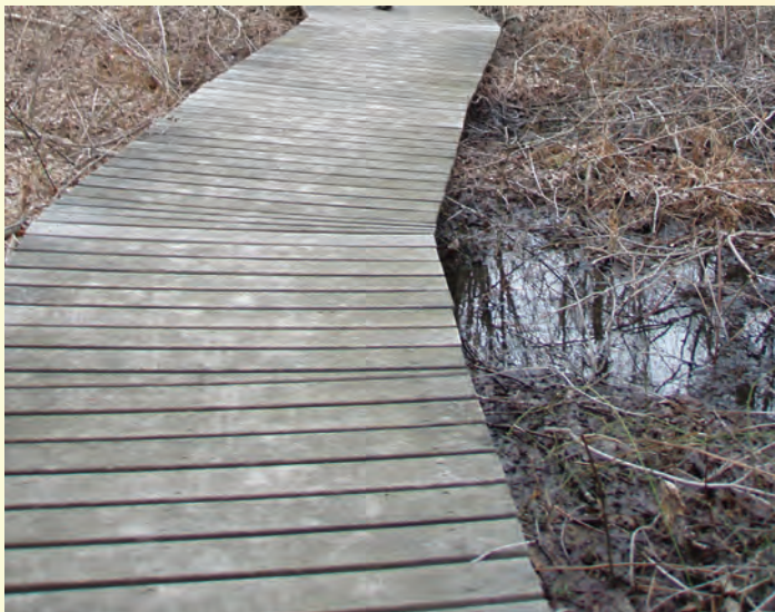
Wet areas in lowlands where streams cross the trail need a bridge or boardwalk
